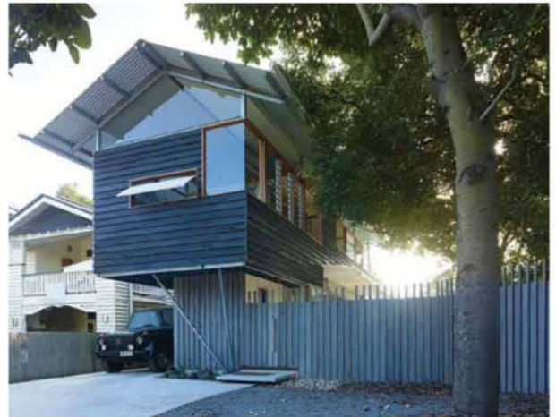
Chelmer House and Studio was designed around the roots of neighbouring trees to take advantage of a leafy outlook.
